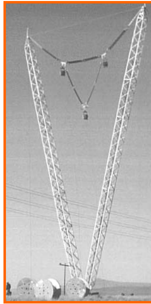
Plate 2.2: Example of compact cross rope suspension tower types
